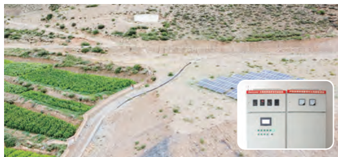
145kW Controllers: 3*PDS33-4T037 + 1*PDS33-4T015 Location: Sichuan Province, China
