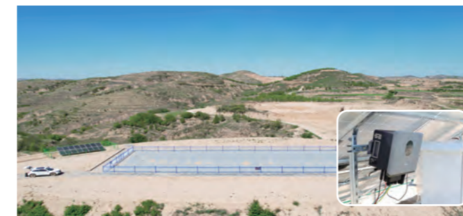
4.8kW Controller: 1*PDS51-4T2R2-E Location: Shanxi Province, China
